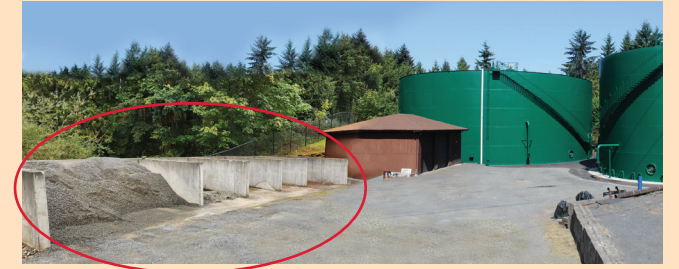
Site of the future Decant Facility
